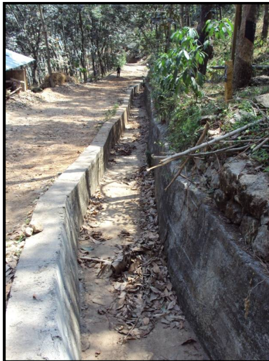
Photographs showing garland drains within project sites to channelize storm water
