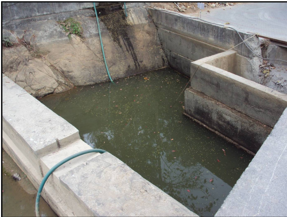
Photographs showing de-siltation trap (Check dam like)
