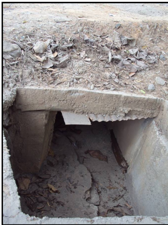
Photographs showing garland drains within the project sites to channelize storm water
