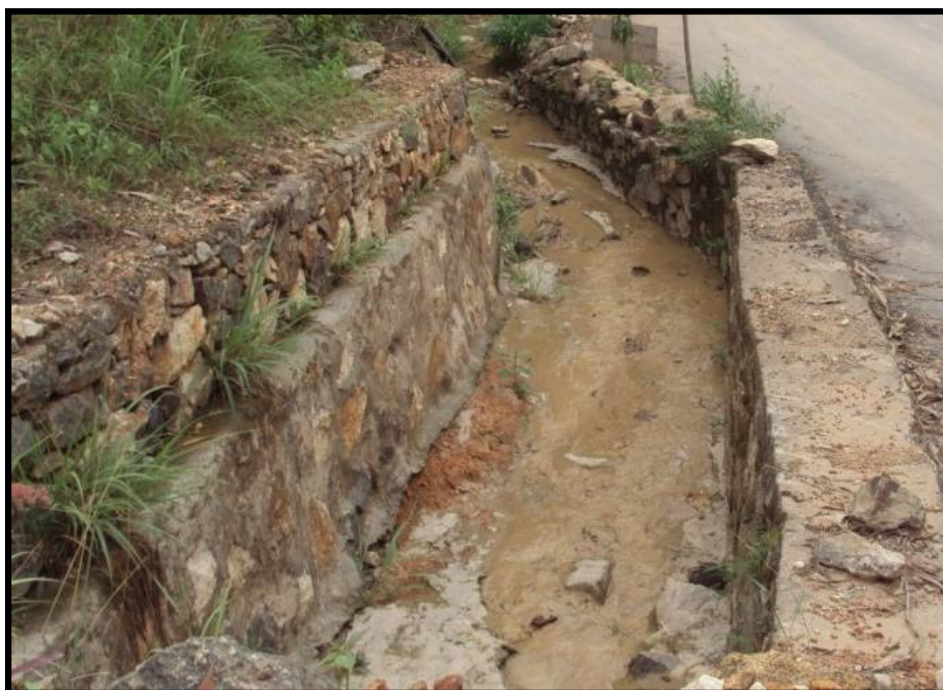
Photographs showing garland drains within the project sites to channelize storm water
