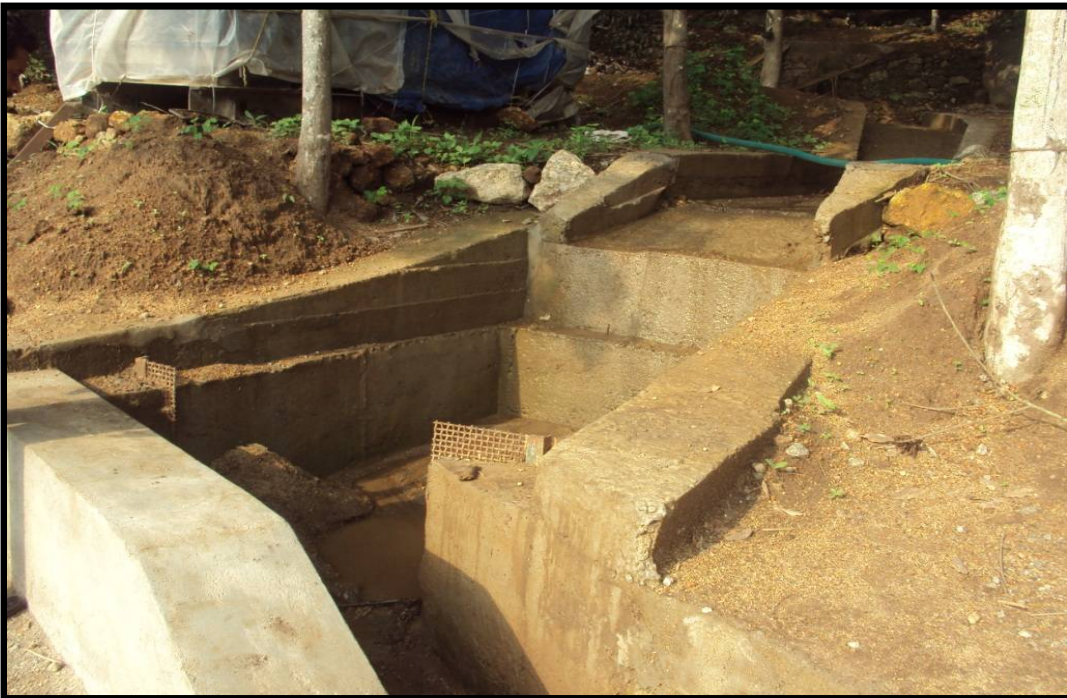
Photographs showing garland drains within project sites to channelize storm water
