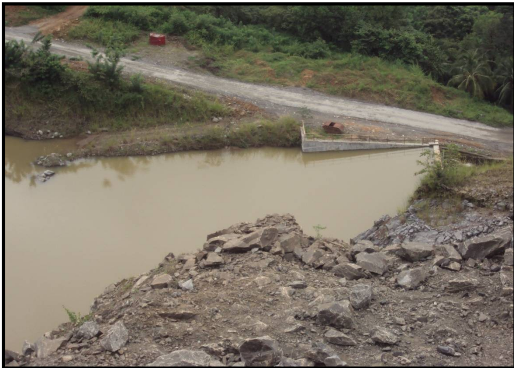
Photographs showing the storm water collecting pit
