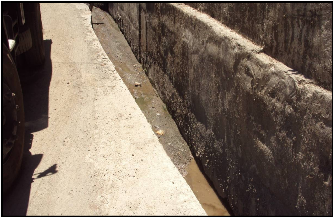
Photographs showing garland drains to channelize storm water
