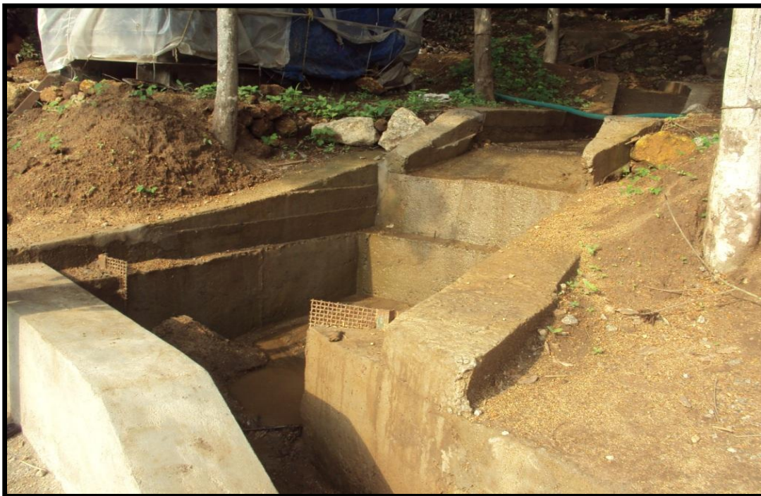
Photographs showing garland drains within project sites to channelize storm water
