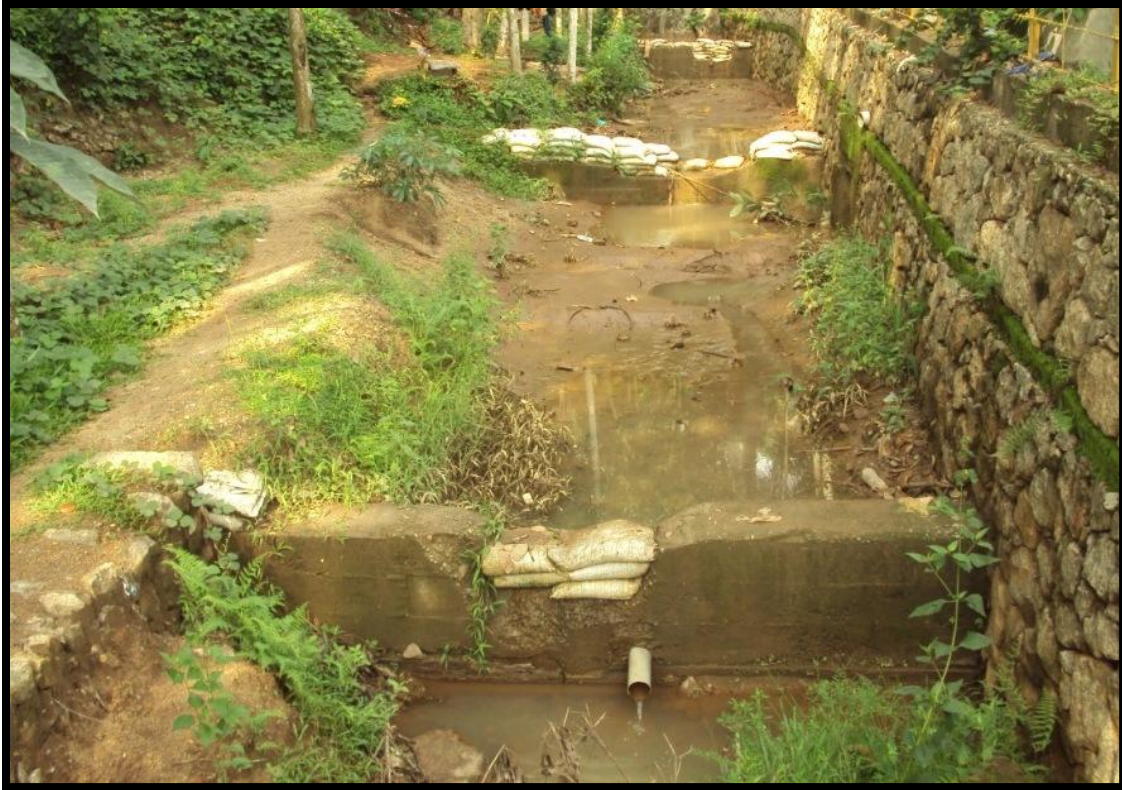
Photographs showing storm water channels with de-siltation trap (Check dam like)
