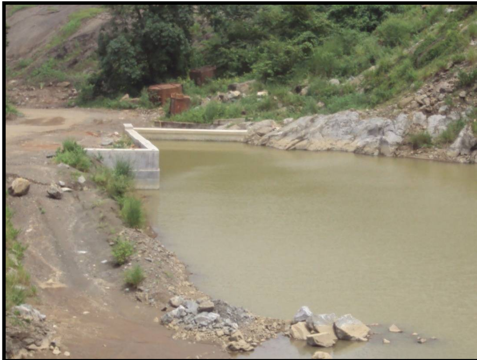
Photographs showing the storm water collecting pit
