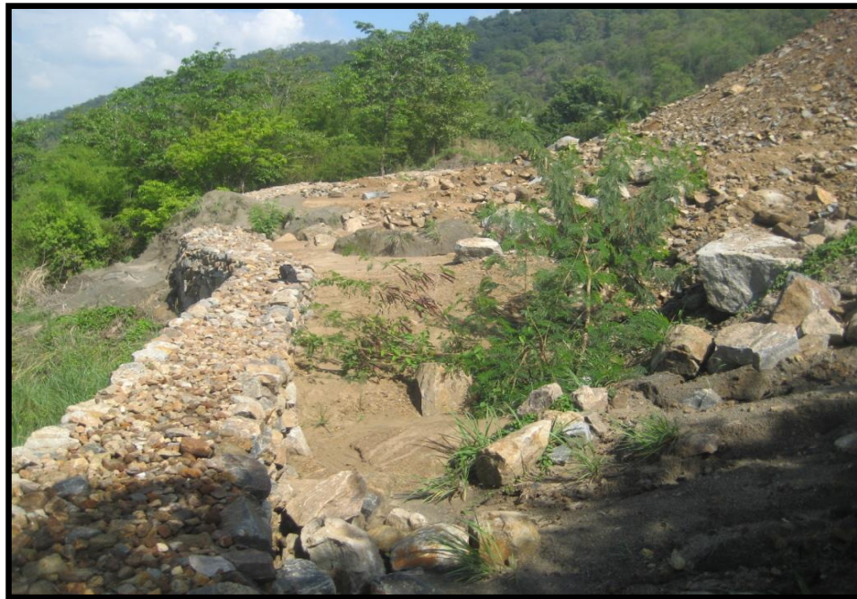
Photographs showing the protective walls at the foot hills to prevent soil erosion
