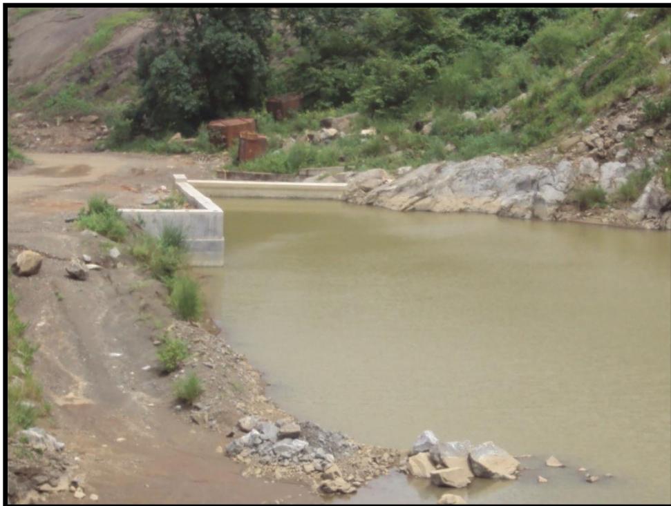
Photographs showing the storm water collecting pit
