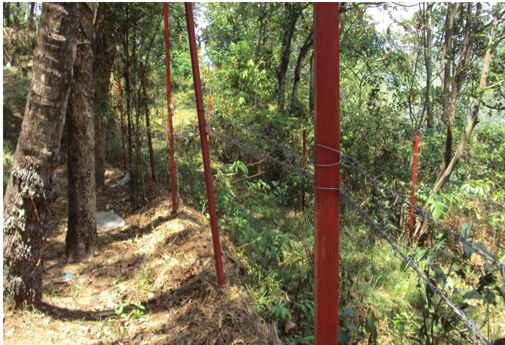
Photographs showing the barbed metal wire fencing installed around the mining area
