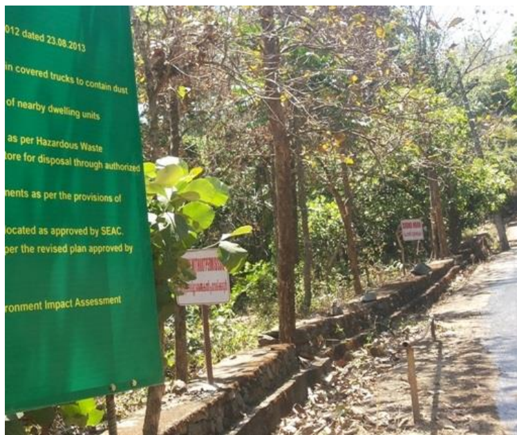
A photograph showing the Garland drains in the project area
