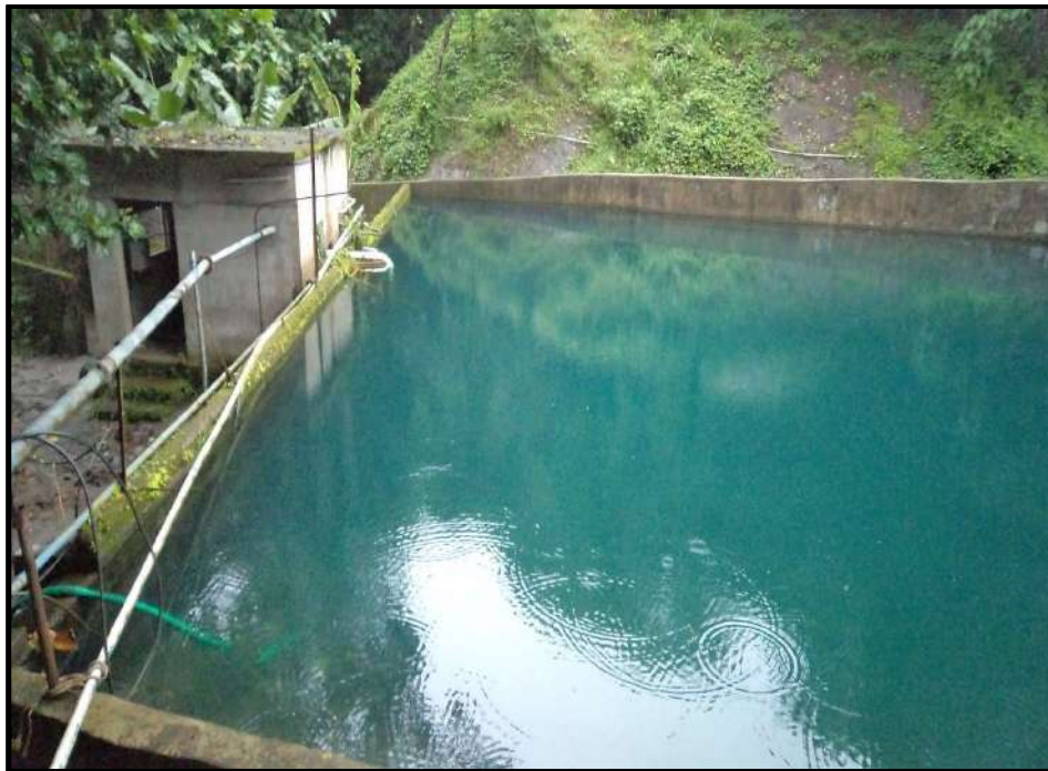
Photograph showing the excavated pit and concrete tank using as rainwater harvesting system
