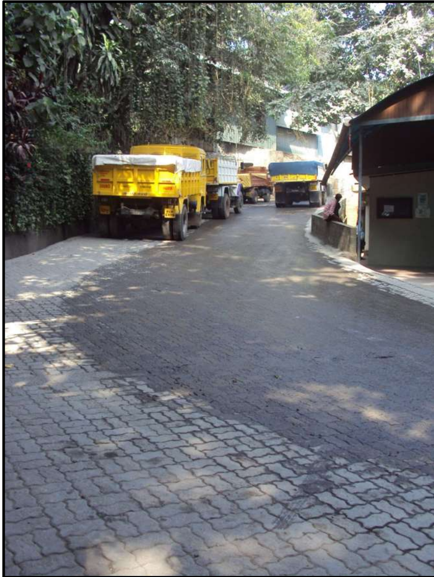
Photograph showing access road constructed with concrete bricks
