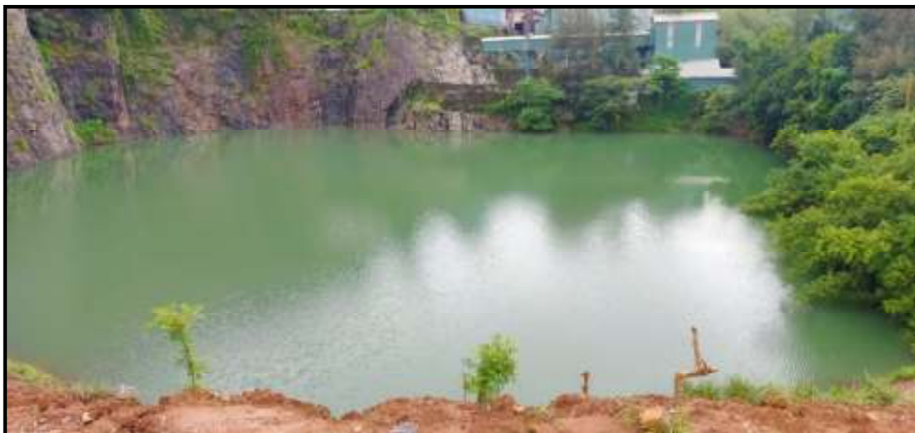
Photograph showing abandoned Mined out pit using as rainwater storage system
