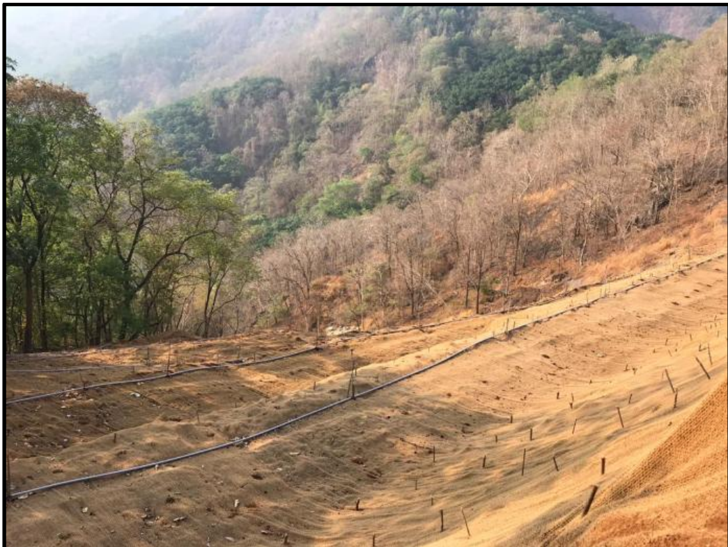
Photograph showing the Overburden/topsoil dump stabilized by geotextiles and vegetation
