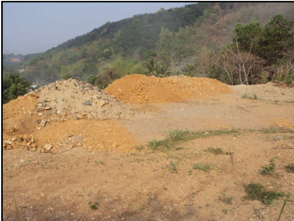
Photograph showing the stacked overburden and top soil
