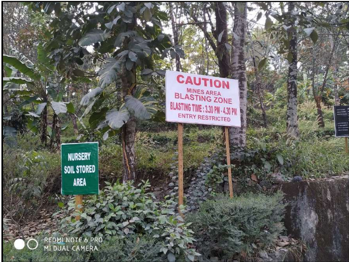
Photograph showing the danger board indicating blasting time installed in the project site
