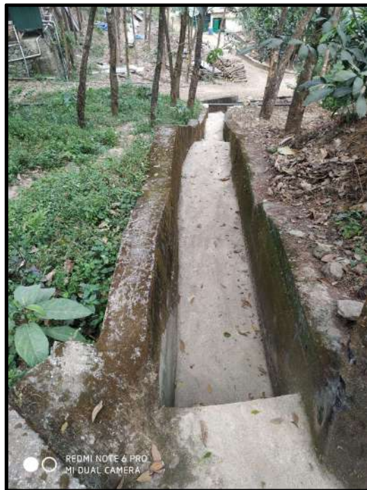
Photographs showing storm water channels with de-siltation trap (Check dam like)
