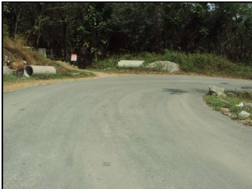
Photograph showing the tarred Access road to the quarry
