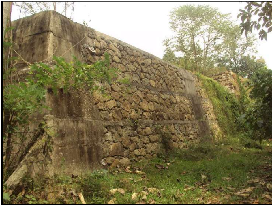
Photographs showing top soil storage area
