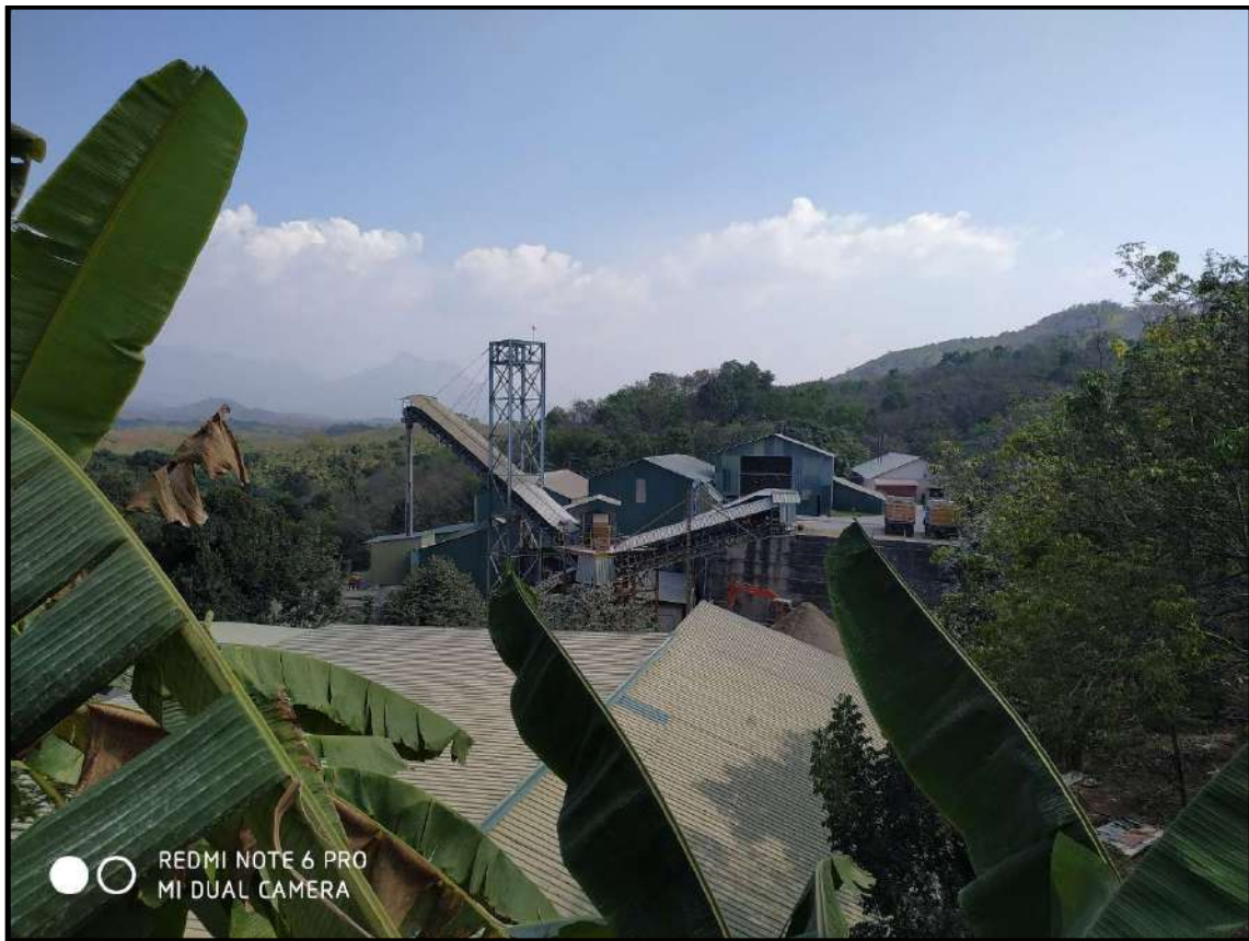
Photograph showing the crusher unit covered by thick green belt and metal sheet envelop
