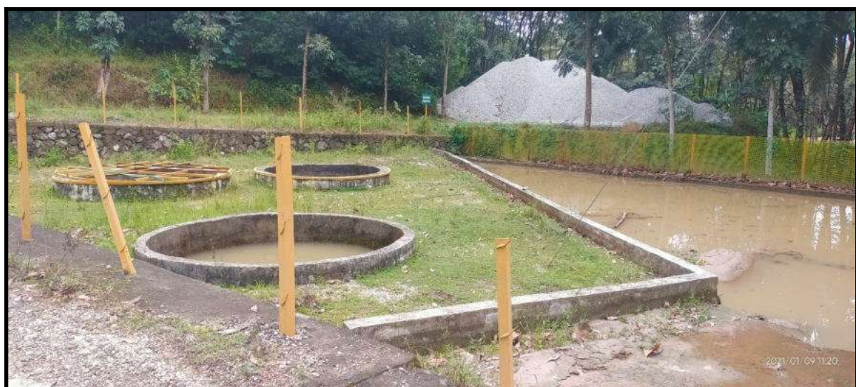
Photographs showing the rainwater harvesting system in the project area
