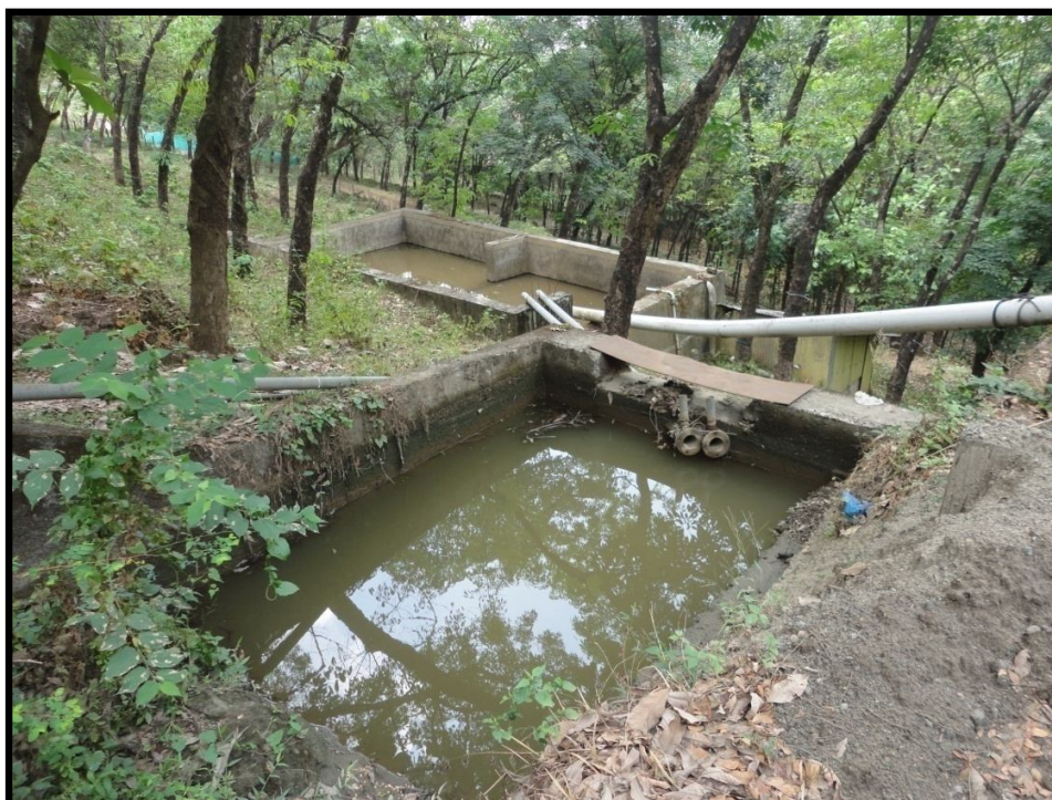
Photograph showing Garland drains with silt/debris trap and desiltation tank
