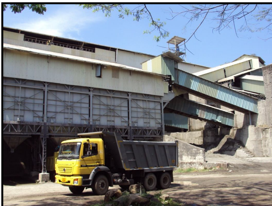
The photographs showing the crusher unit encircled by green belt, hollow brick envelope and metal sheet envelop
