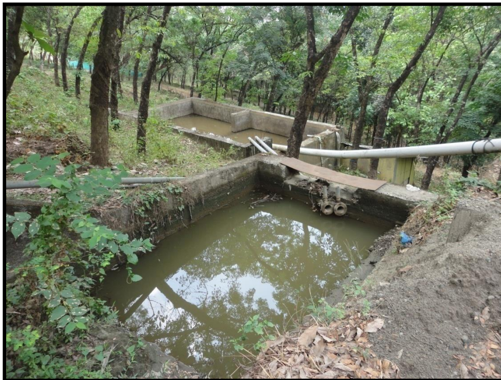
Photograph showing Garland drains with silt/debris trap and desiltation tank
