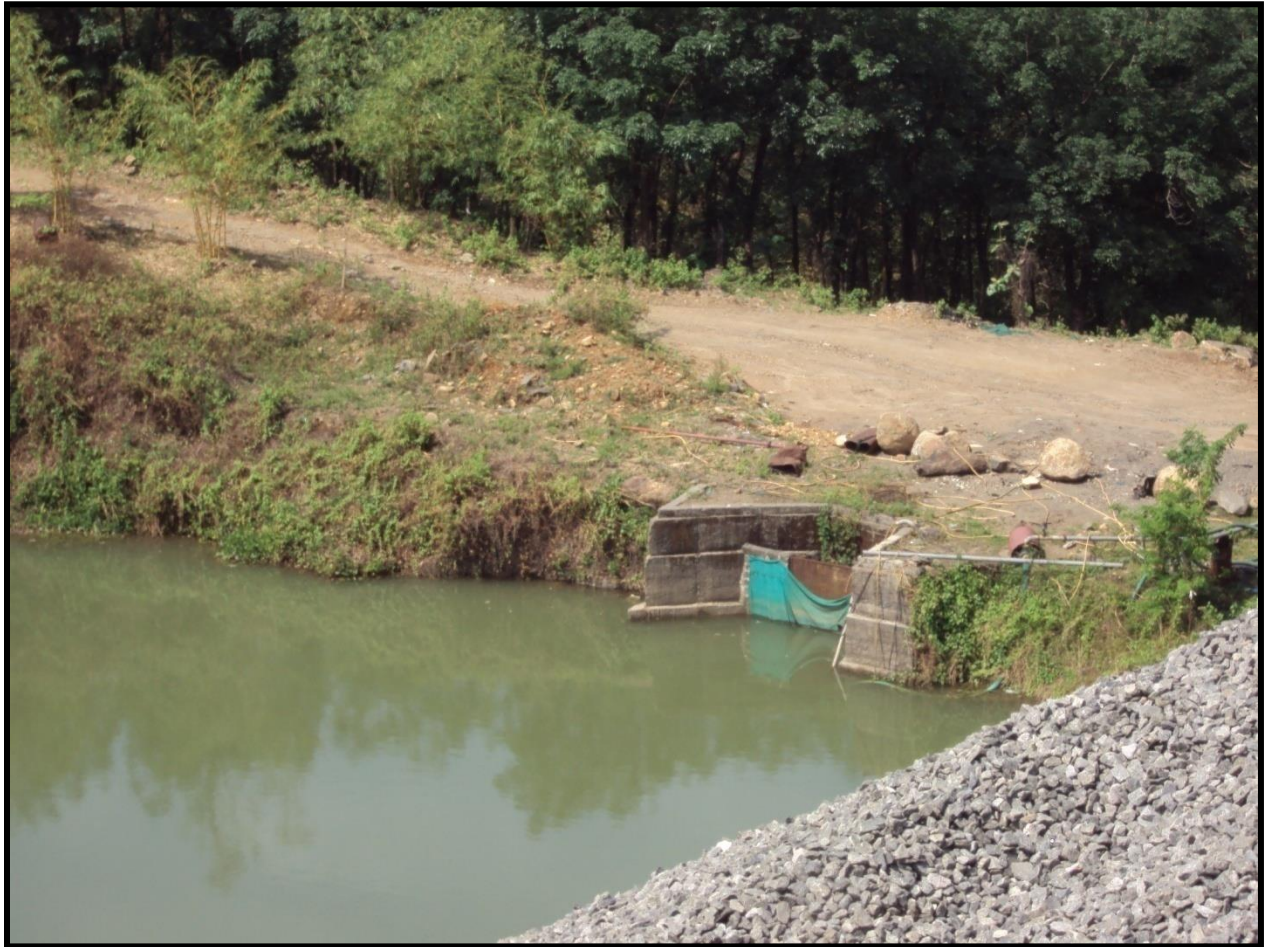
Photograph showing opening of storm water collecting pit guarded with net trap
