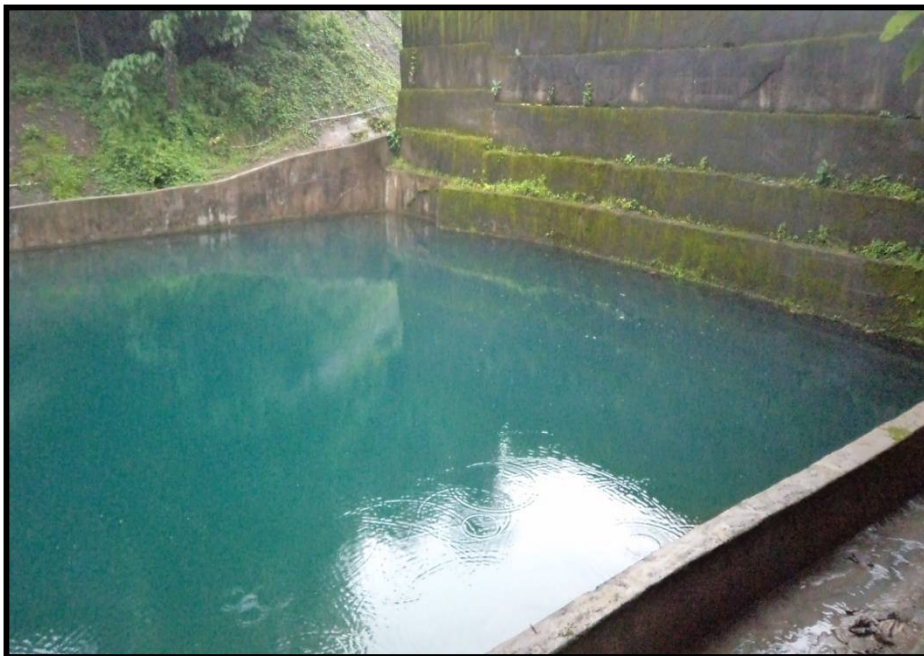
Photograph showing the excavated pit and concrete tank using as rainwater harvesting system
